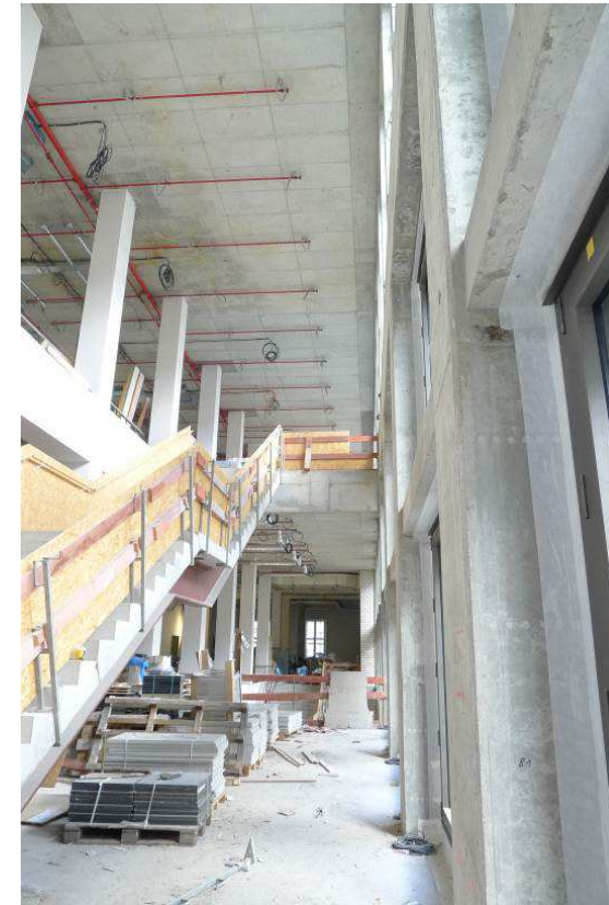
Fig. 11: View into the staircase hall, construction site, Photo BBR, July 2017
